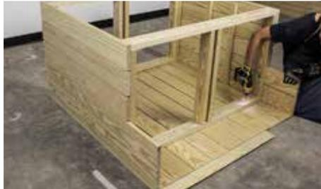
Flip assembly if desired and evenly space the remaining Parts (B) and attach to both frames. The spacing should be close to 1/4", but measure your stock.
