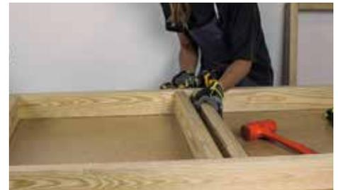
Place two Parts (E) inside the rectangle so they are centered and spaced  $\frac{7}{8}$ " apart from each other. Use a mallet if needed. Secure with two  $2 \frac{1}{2}$ " screws.
