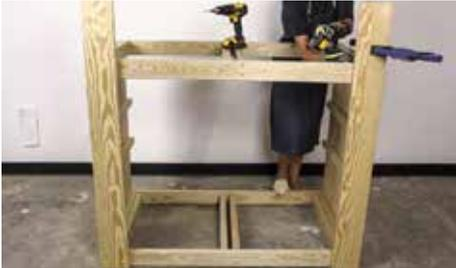
Attach the first Parts (B) to either end of the bar, securing from the frame side if visible screw heads are not desired. Use four 2" screws per board.
