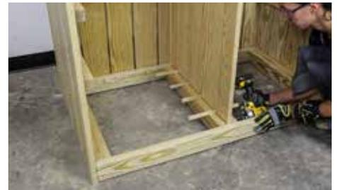
Finish by securing the bottoms of Parts (F) and (G) to the bottom frame.
