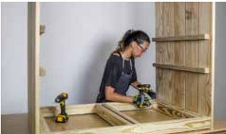
Next, flip the second frame on the work surface and attach the side walls using four  $3\frac{1}{2}$ " screws per board.
