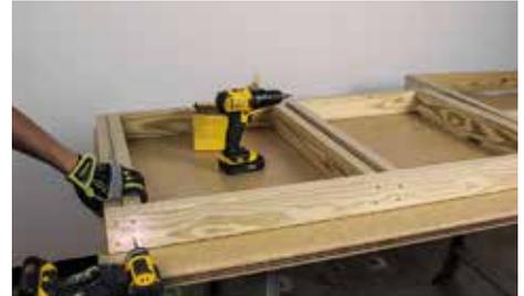
Repeat this on the other short end and secure to the frame with two  $2\frac{1}{2}$ " screws.
