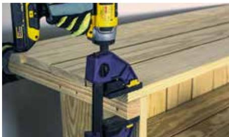
Attach the first and last board with two 1 1/4" screws per board, avoiding the screws perpendicular in the support pieces.
