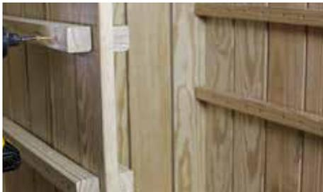
Using the marks as guides, secure the opposite Parts (C) so that they avoid the screws on the other side. Use the same method of finding level to its mirrored side with a spare Part (N).
