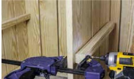
Using the line as a guide, clamp and secure Part (C) to the middle wall using two 2" screws per board.
