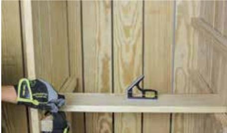
Using a level, place a Part (N) perpendicularly on top of a Part (C), and move Part (C) up and down until the level bubble is in the middle. Mark a line above Part (C) with a pencil.
