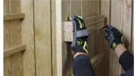
Repeat Steps 25-26 for the upper Part (C), and then place another Part (C) on top of both secured pieces and pencil-mark screw hole guides in between the ones you made.
