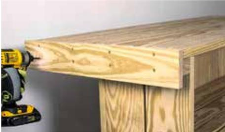
Attach apron Parts (M) and (L) to the outside edges with two 1 1/4" screws vertically placed to complete the bar top.
