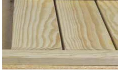
Ensuring that the total length of the boards plus spacers equals  $27 \frac{1}{4}$ ", block up the bottom edges and secure boards with a clamp.
