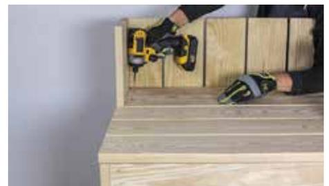
Secure Parts (I) to complete the countertop. Once complete, check that the bar is level on the ground. Use shims under the protruding 2x4s on the base frame as needed.
