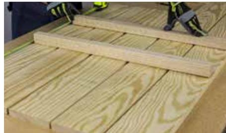
Lay the second Part (C)  $25 \frac{5}{8}$ " from the bottom edges.
