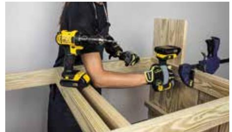
Continue securing the top frame until all boards are joined.
