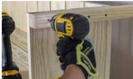
Add support Parts (J) to the outside of Parts (B) with two 2" screws per board.
