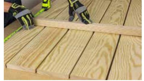
Lay a Part (C)  $16 \frac{1}{8}$ " from the bottom edges. Measure and mark both ends to draw a pencil line.
