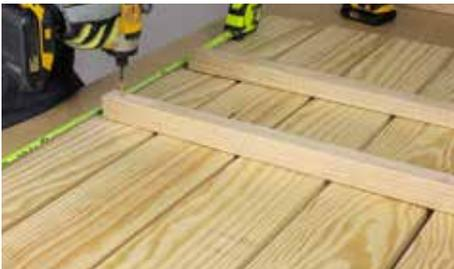
Secure Part (C) to the boards with two 2" screws per board.
