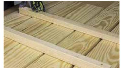
Secure Part (C) to the board with two 2" screws per board.
