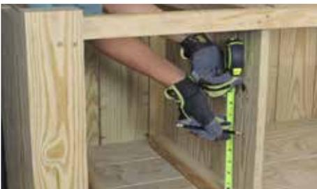
Measure and mark a line on Parts (K) that is 5 1/2" up from the Part (C) as shown.
