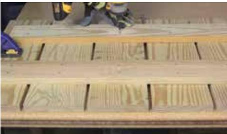
Build the longer, right side door using five Parts (I) and one Part (J), plus two Parts (S) as battens. Use 1/4" spacers and attach with two pairs of 1 1/4" screws per board. Dry fit assembly before attaching all screws.
