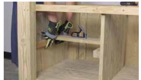
Lay a Part (K) on top of another Part (C) and, using a level on top of (K), slide Part (C) until it is level with its mate on the other side. Mark the line, remove Part (K), and secure Part (C) using four 2" screws.
