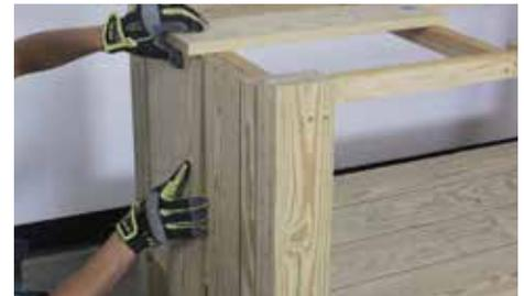
After attaching the other Part (H) to the right side, continue attaching Parts (I) using two sets of three 1" nails. Use a Part (N) to ensure the top is flush.
