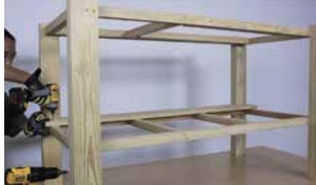
Secure Part (F) to the frame using 1 5/8" screws. Secure the two edges and then fill in the middle screws. Use two 1 5/8" screws per 2x2 frame support.
