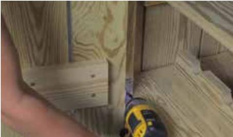
Secure the door hinges to the front legs using the hardware provided in the hinges. Test both doors and ensure they open and close smoothly.
