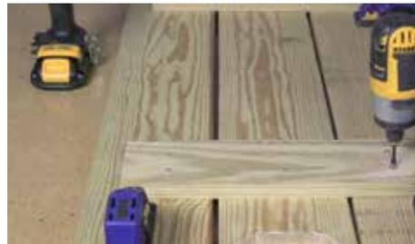
To make the lid, assemble Parts (R) where the detail cut piece is in the middle and Parts (Q) are on top, 3 1/2" from the edges. Use 1/4" spacers, and attach Parts (Q) using two pairs of 1 1/4" screws per board.
