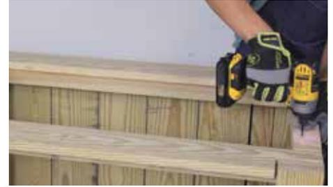
Cap the right side with three Parts (P) evenly spaced. Use two 1 5/8" screws per board.
