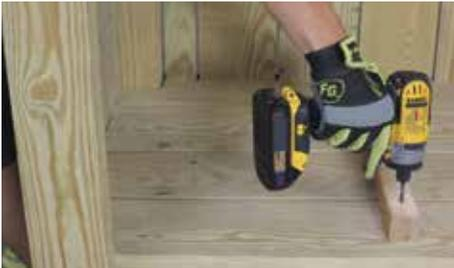
Place a Part (C) on the outside of this line, where it is 3" from the back wall. It should be directly below the Part (C) above. Secure with two 2" screws per board.
