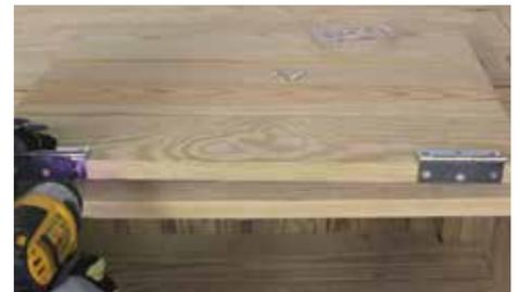
Add hinges 1" from each edge to the front of the doors as shown. Note that when looking at the front of the doors, Part (J) should be on the right of the big door and on the left for the small door. Dry-fit before completing.
