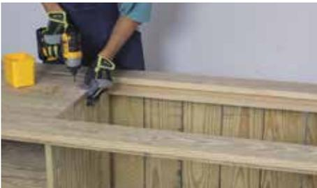
Next, attach Parts (O) in between Parts (N), evenly spacing and securing with four 1 5/8" screws per board.
