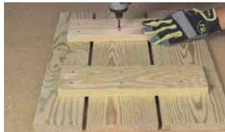
Build the left door in the same manner, using two Parts (I) and one Part (J) with Parts (T) as battens.
