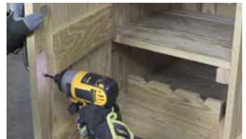
Attach the handles to the front of the doors so they are 2" from the top of the door and 1" from the edge. Use the hardware provided.
