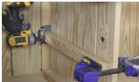
Place a Part (C) above this line, clamp, and secure with four 2" screws to Part (K).
