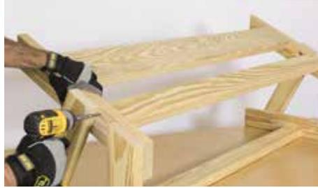
Flip the assembly over and attach another Part (E) so that it is 3 1/4" from the top of Part (C). Secure Part (F) on this side so it is 2 3/4" from Part (E). Use two 2 1/2" screws per side. Repeat until you have created the second bench frame.
