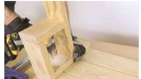
Lay out three Parts (H) with 1/4" spacers in between and apply a clamp to the ends. Place an arm assembly 2 5/8" from the ends of Part (H) and 1/8" from the top Part (H)\*. Clamp as needed and secure with six 2" screws.
