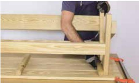
Place a bench frame upside down on top of the bench seat you just made. Center the frame on the seat. Slide a Part (G) on the inside of the frame and attach to Parts (H) with two 2" screws per board.
