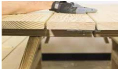
When placed together, the backrests continue the  $\frac{1}{4}$ " spacing through the table top. Add another bolt pair on the other end to complete the assembly.
