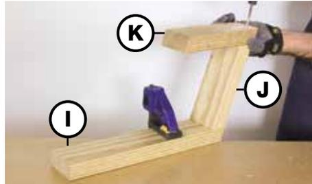
Next, flip the component so that Part (I) is on the work surface, and attach Part (K) in the same manner.
