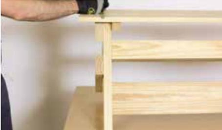
Orient a bench so that the angled leg is facing you. Then measure and mark a line  $9 \frac{5}{8}$ " from the front lip of the seat as shown. Do this on both ends of the bench seat.
