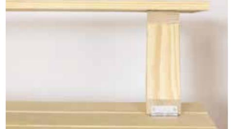
Secure just the middle screw on the top and bottom of the hinges first.
