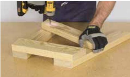
Place Part (D) 9" down from bottom right edge of Part (A) and secure one end.
